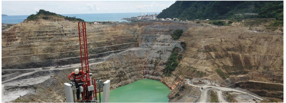
Private cellular network alleviates safety concerns by keeping networking gear and technicians out of the pit.
